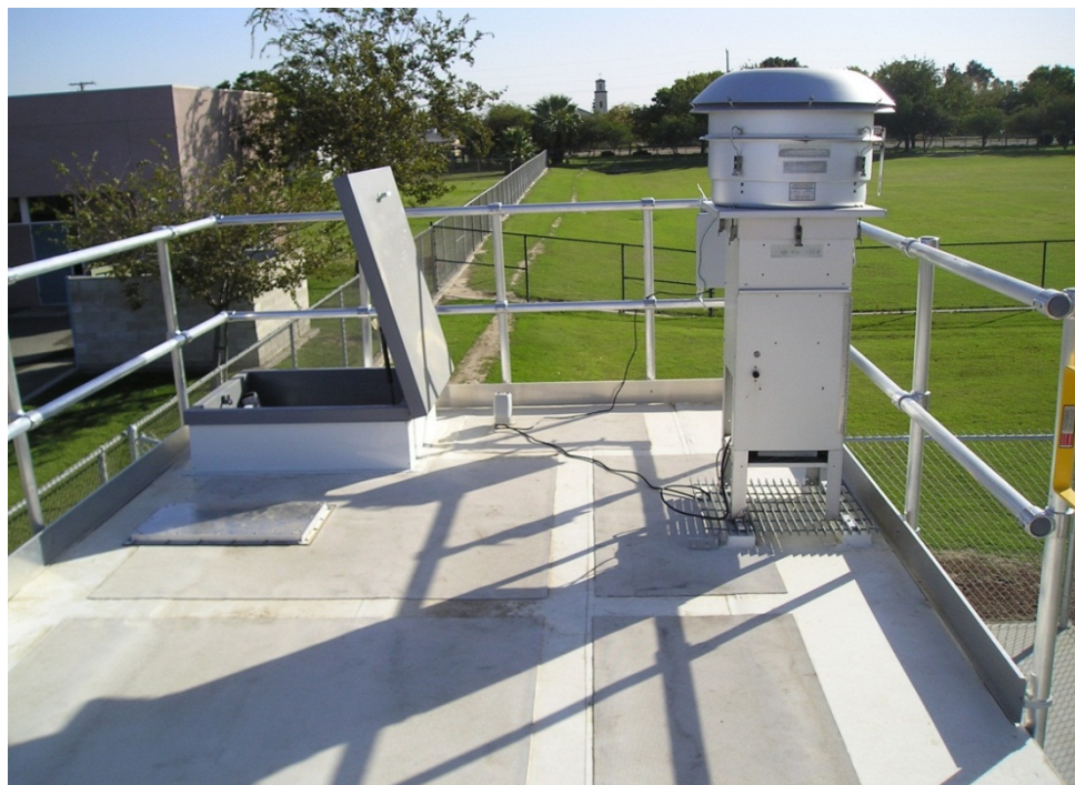
Roof platform with roof hatch, safety railing, non-slip walkway, and toe kick
