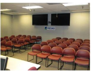
There are two pairs of 65" Sharp Aquos monitors in the front and rear of the room each connected to a Crestron DM-RMC-SCALER-C. There are two Sony EVI-HD1 people cameras to provide video coverage from the front and rear of the room. There is also a fixed ceiling-mounted Wolf Vision EYE-10 document camera. Room system controlled by Crestron CEN-COM boxes and a Crestron V15-TILT-B control panel with custom-designed layouts.
