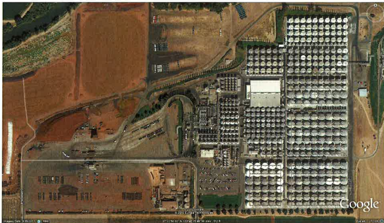
Figure 3. Existing Winery Facility
