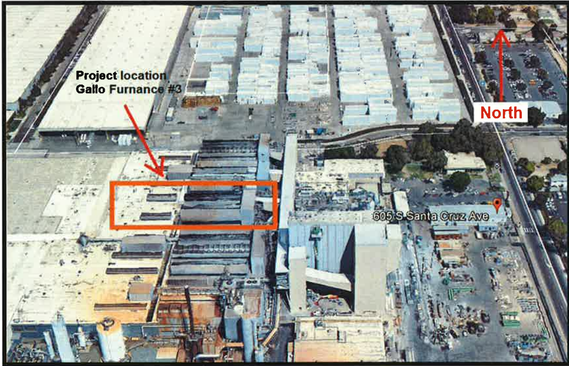
Figure 7: Gallo Glass Company Project Site View to North
