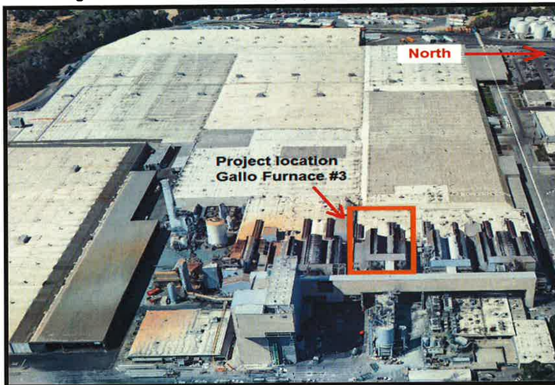
Figure 10: Gallo Glass Company Project Site View to West
