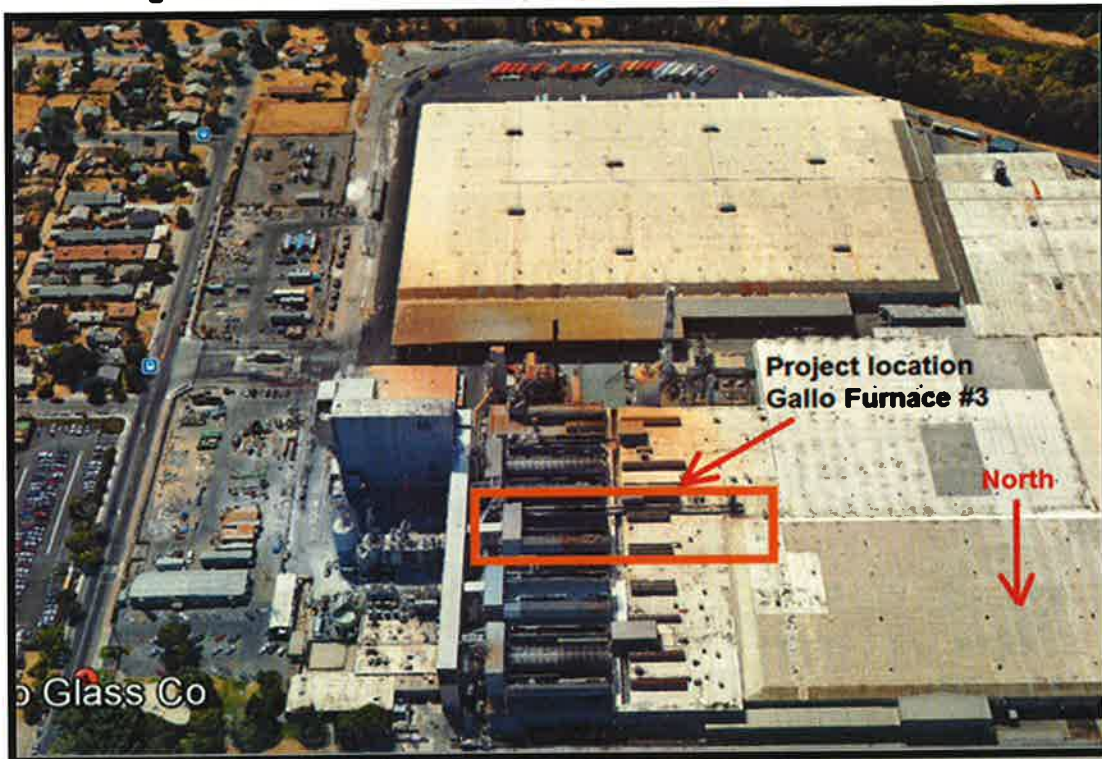
Figure 8: Gallo Glass Company Project Site View to South
