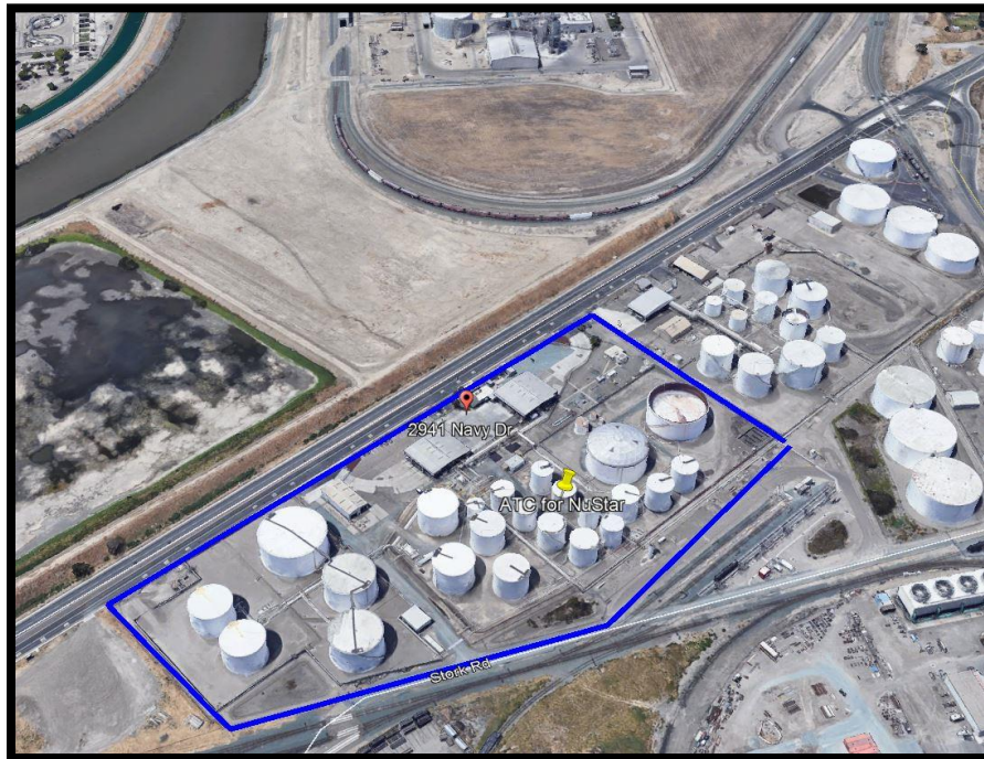
Figure 9: NuStar Modification view to the West
