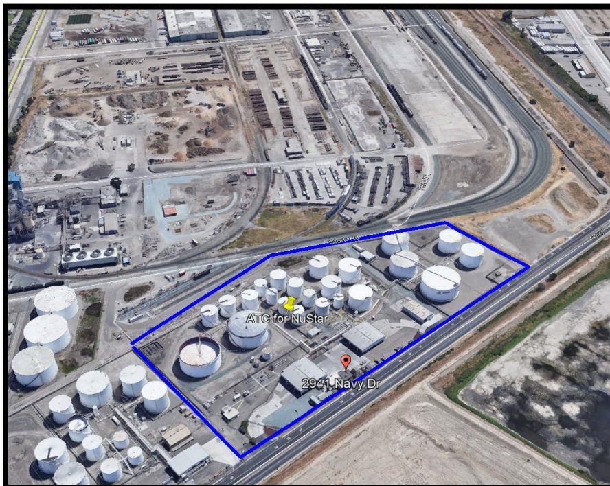
Figure 8: NuStar Modification view to the East
