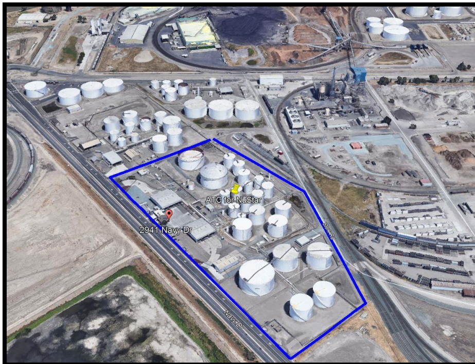
Figure 6: NuStar Modification view to the North
