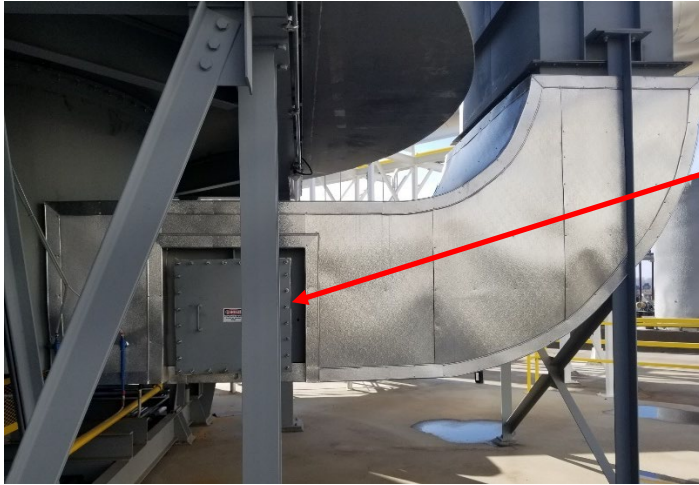
Figure OMP-1A RTO Odor Sample Port Location
