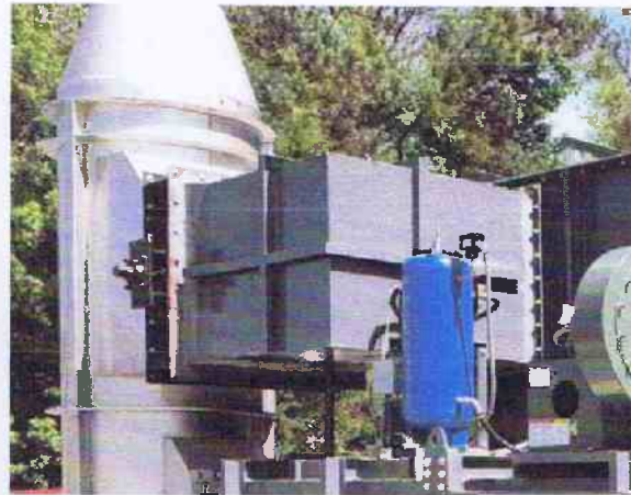
Typical Hot Gas By-Pass Damper Assembly
