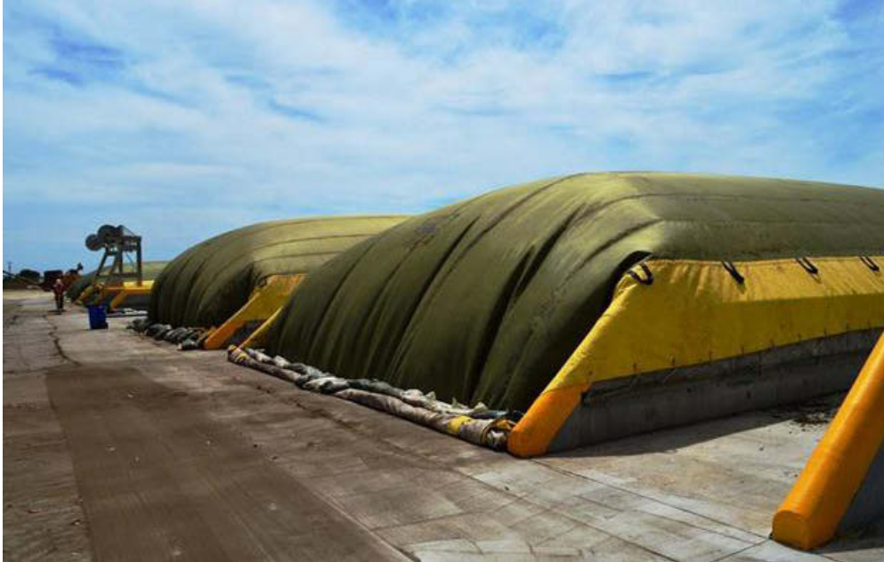
Source: Cal Recycle Blog – Gore® covers utilized on composting operation at Mid Valley Disposal
