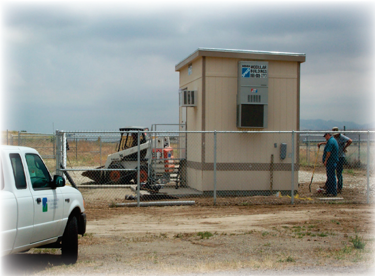
Building is set in place to hold air monitoring equipment.
