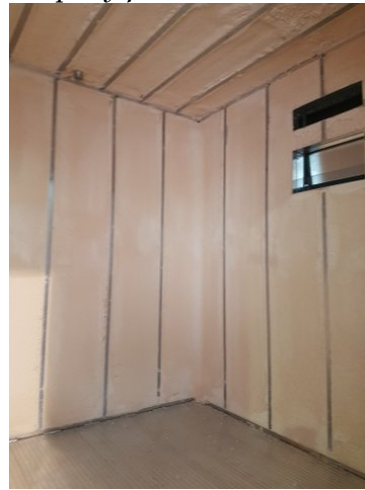
Spray foam Insulation
